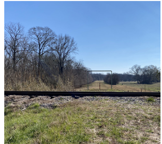
EXISTING: The levee trail at Carolyn Crayton Park intersects with railroad tracks and extends onto private land.
