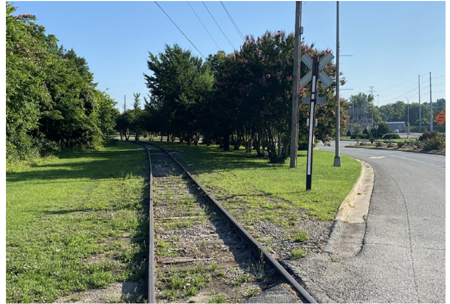
EXISTING: Riverside-Walnut railroad spur; north view
