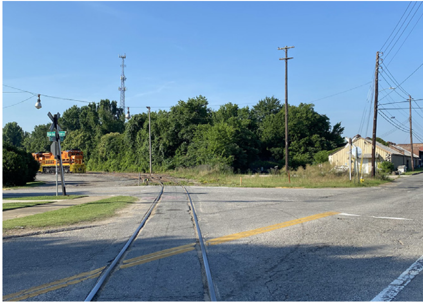
EXISTING: Riverside-Walnut railroad spur; south view
