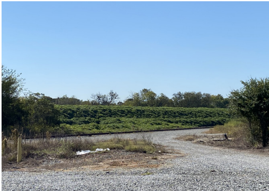
EXISTING: Raised rail ramp
